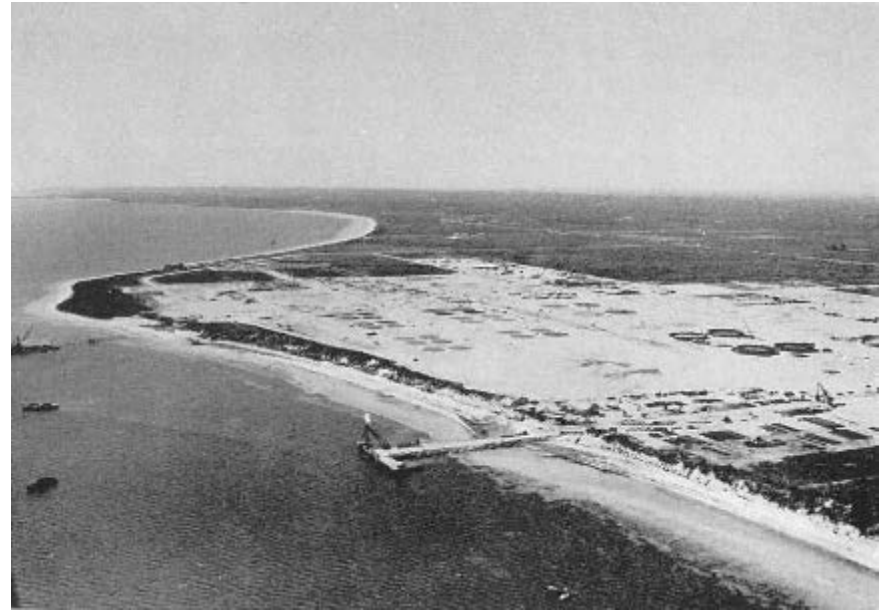
Beginning of the Oil Refinery Work 1953 Source: BP Developments Australia
