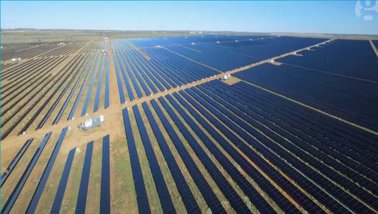
Broken Hill solar farm.
