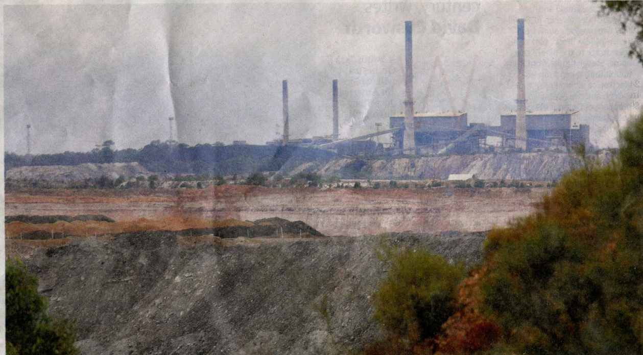
Synergy's coal-fired power stations have been running below capacity because of green power surges. Picture: Sharon Smith
