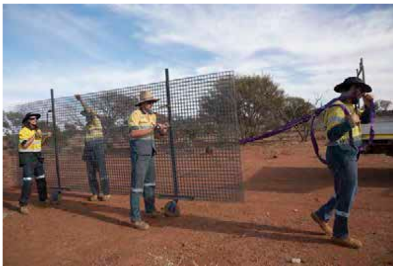
Mesh carrying jig developed by GCo to transport MWA ground plane material long distances on foot. Image Credit: Curtin University
