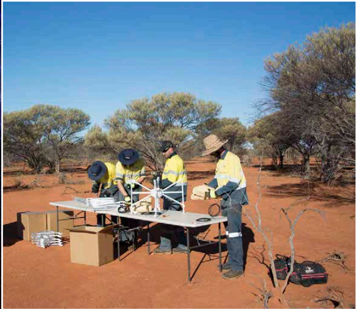
Portable production line for assembling MWA dipole antennas at each remote tile location. Image Credit: Curtin University
