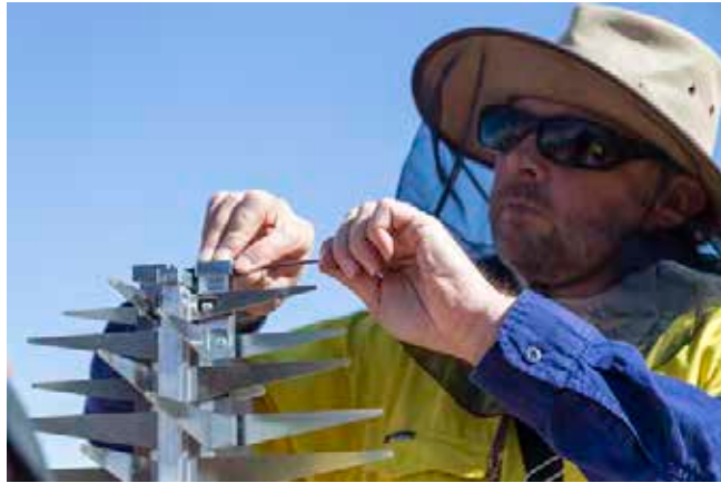
Figure 7, left: Commissioning the amplifiers on top of the SKALA4.1 antennas. Credit: ICRAR, 2019
