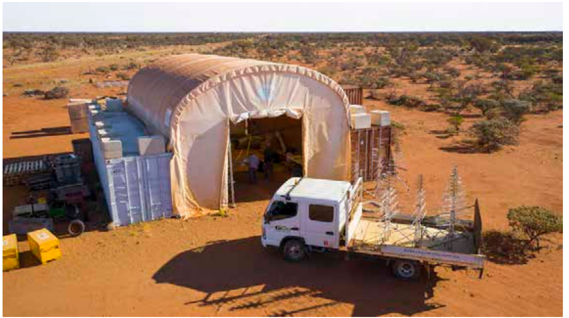
Figure 6, above: Aerial view of the dome shelter on site, where the antennas for SKA Low stations were constructed. Credit: ICRAR, 2019
