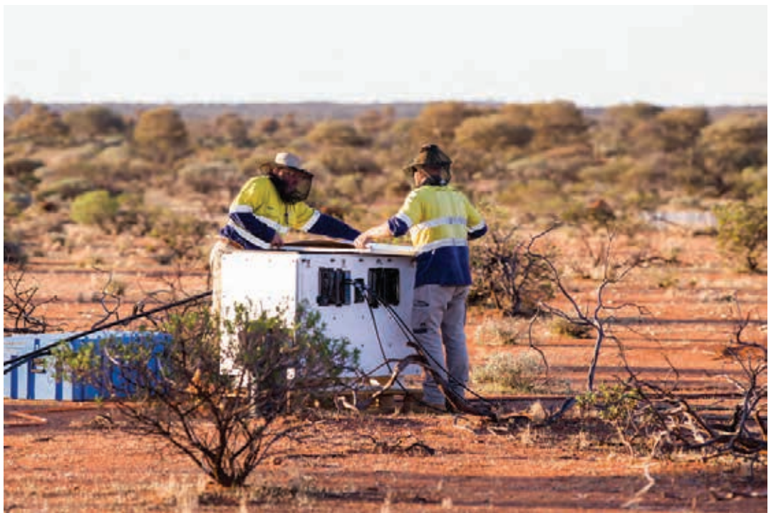
Figure 2, above: Avoiding the flies as we put the cover on a temporary cable housing box. Credit: ICRAR, 2019
