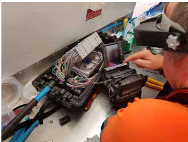
Figure 9, left: Mitchell & Brown testing a fibre splice. Credit: Curtin, 2019
