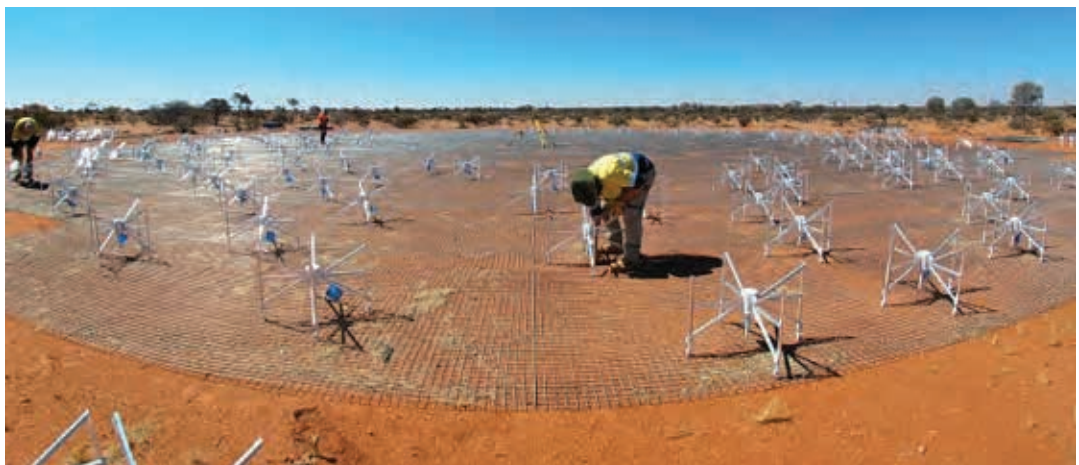
Figure 2, above: EDA2 Dipole antennas being installed on the mesh ground plane. In the middle of the photo is shown the equipment used to accurately survey each dipole location. Credit: Curtin, 2019
