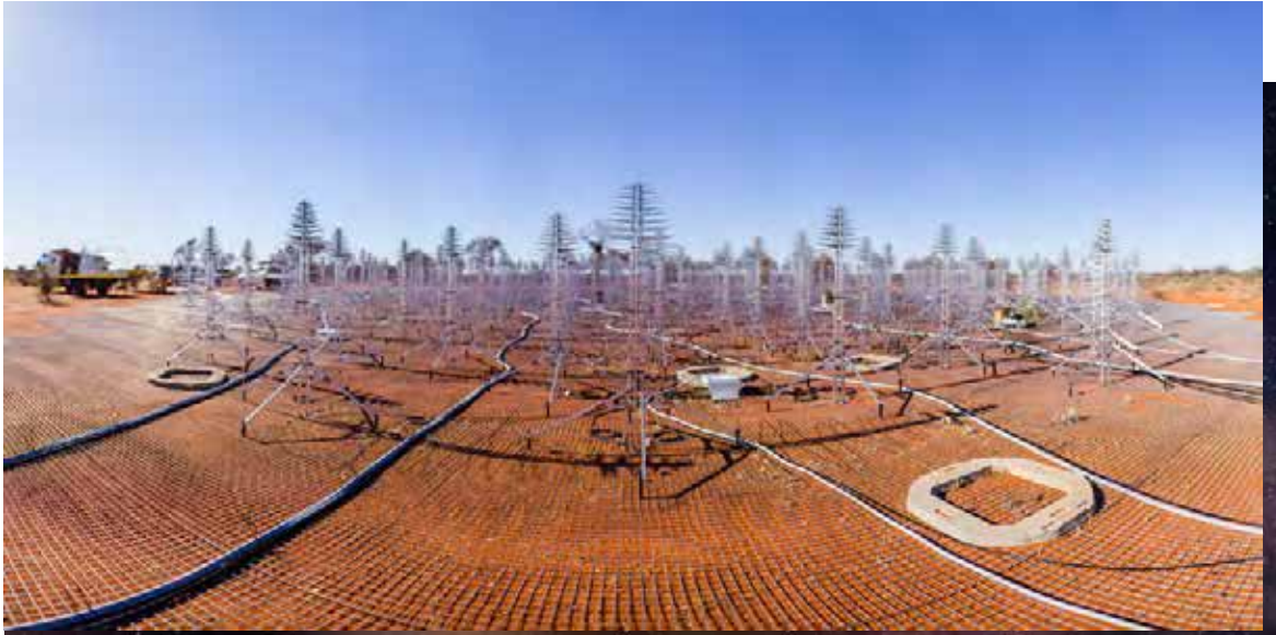
Below: The AAVS2 station, completed in 2019, with 256 'Christmas-tree' antennas. Credit: ICRAR
