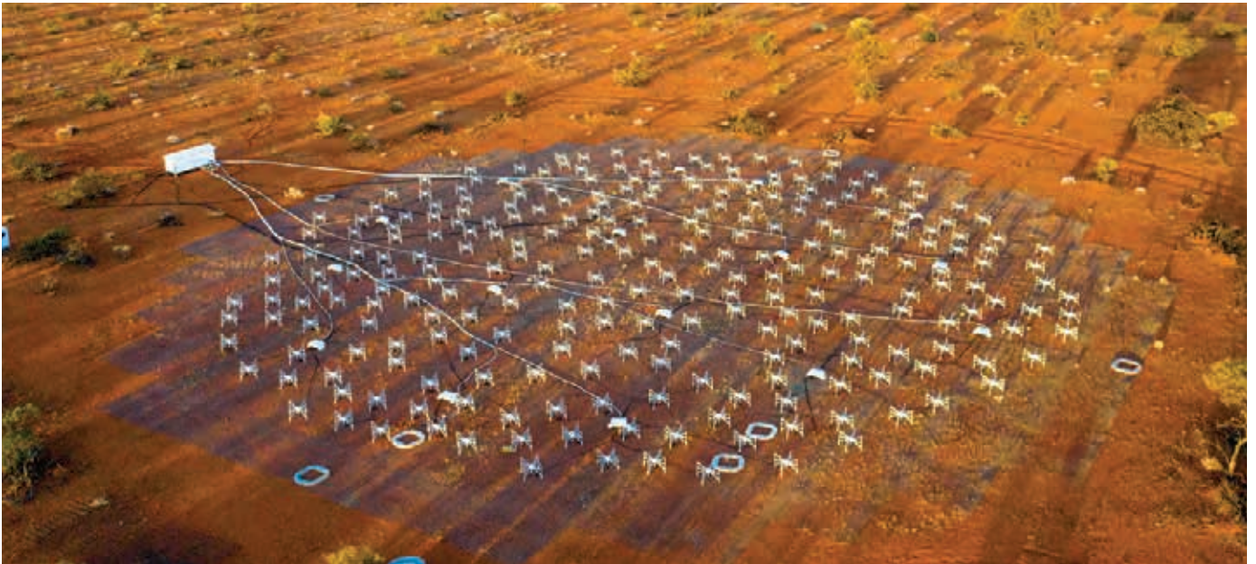
Figure 2, above: Aerial view of the completed EDA2 station. Credit: ICRAR, 2019
